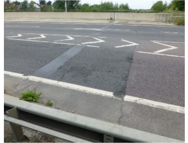
East expansion joint, Westbound carriageway.
